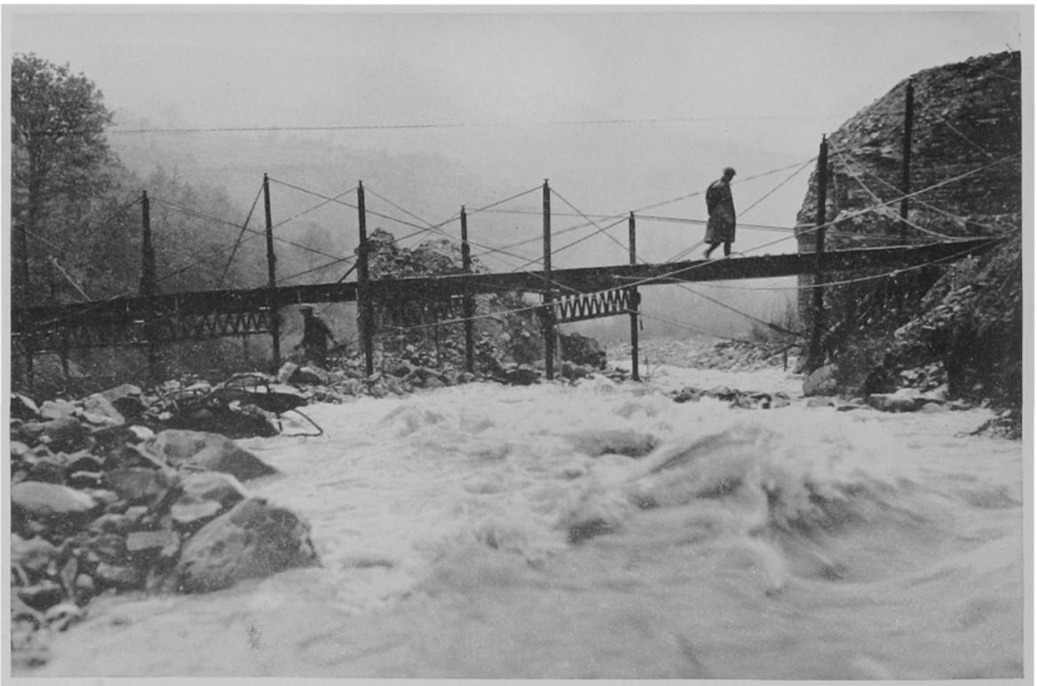
*Engineers prepare to remove a trestle bridge which has been undermined*
